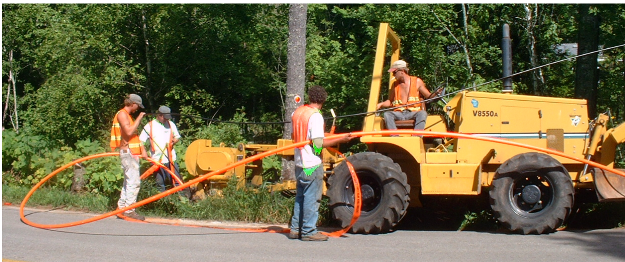
Laying cable in Door County.
