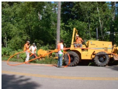
Using a "Ditch Witch," the cable-laying crew installs the orange conduit pipe at the roadside
