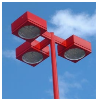
Target's light fixtures minimize light pollution
