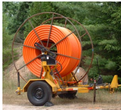
The fiber optic cable will be threaded inside this plastic pipe. This way, should we ever have another upgrade, it can be done without as much disruption and digging
