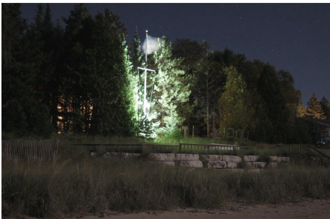
This photo shows some mistakes with the outdoor up-lighting of a flagpole. Being floodlit, light is scattered needlessly. A narrow spotlight would waste less light and energy if the idea is to just light a flag.
